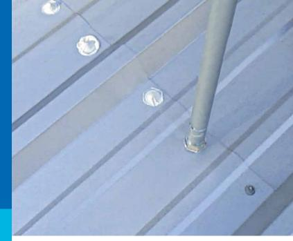
Perfect for covering fasteners, GE Enduris Liquid Flashing is now packaged in foil sausages to use with bulk and special nozzle.
